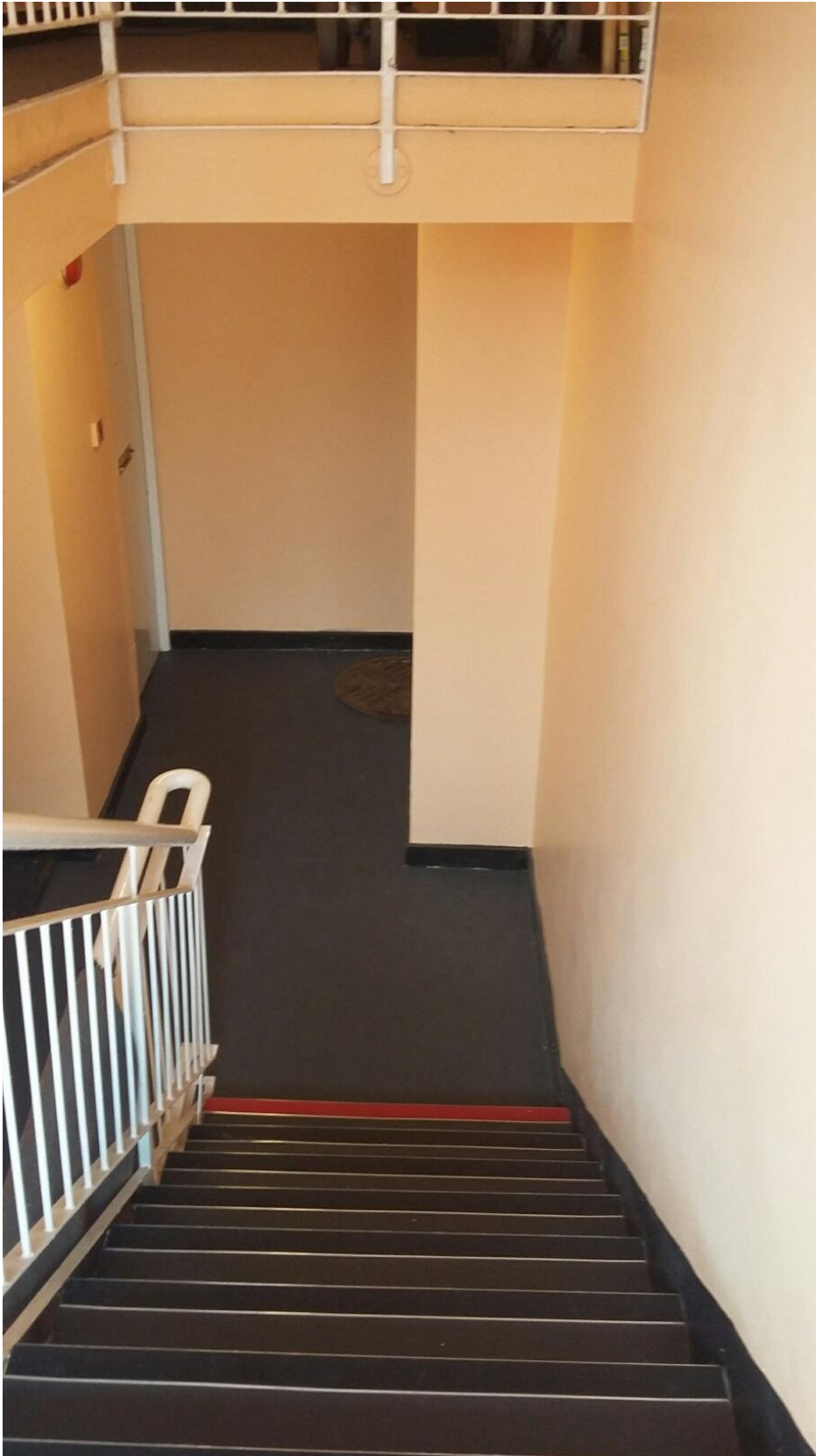
Painting of hallways/stairs, landings and banisters is now complete.
